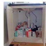
The water damaged area was determine to be directly beneath the left side of the left vanity cabinet of the master bathroom. This was done by referencing the location of the hot water supply pipe and the supply air register in the bathroom floor.
